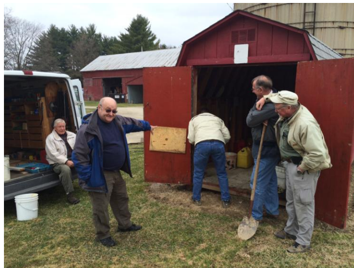
4 th Saturday Crew installing new shed doors
