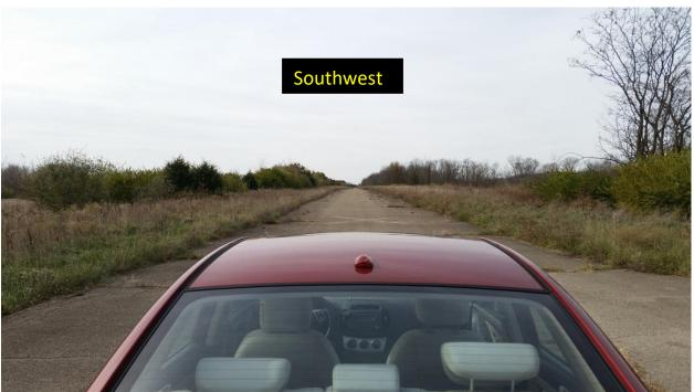
Clearly this runway is not an option for a low winged glider. That said, a high winged aircraft such as 2-33, Piper Cub, Champ, etc may be able to land there safely. A low winged aircraft that has wings well above the ground and/or that bow up, e.g., a Pawnee may also be able to land there safely. I personally would not rule this closed runway out in those type of aircraft if faced with a forced landing situation.
