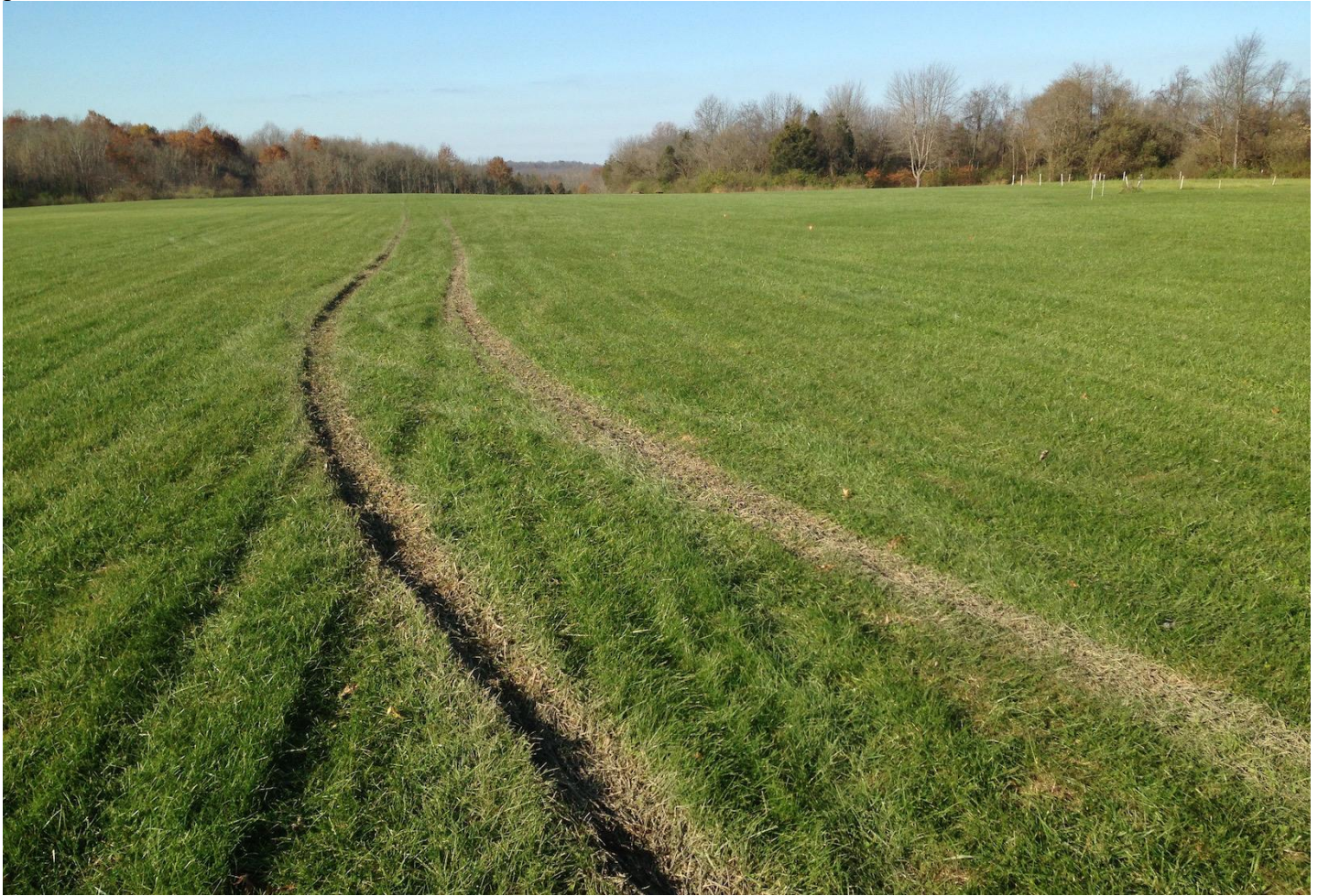
Truck Ruttitis Example - 2017-11-25(Deep truck tire ruts in the middle of the runway.
