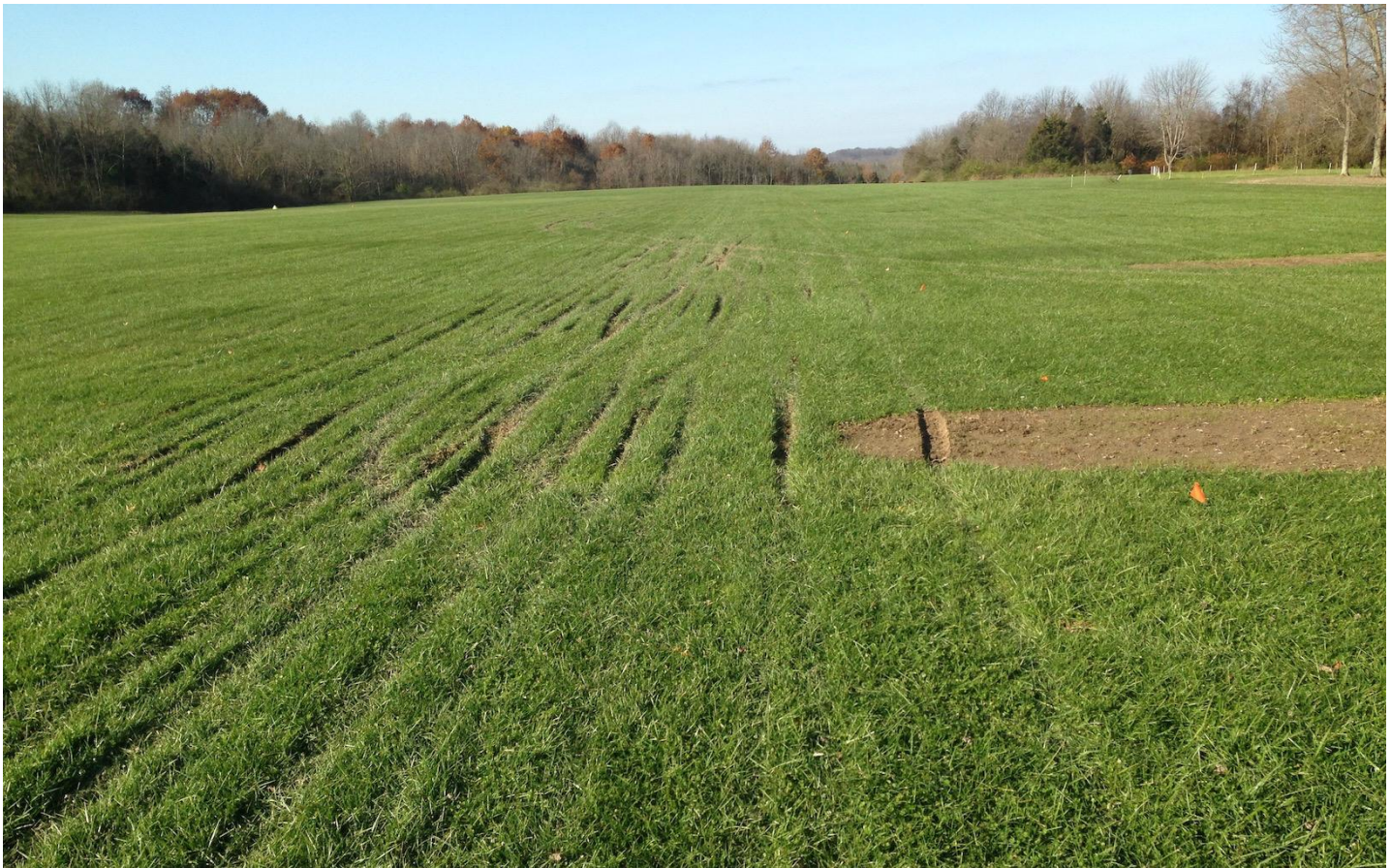
Towplane Rutting Example - 2017-11-25 (Many many deep towplane runs in middle of runway.)
