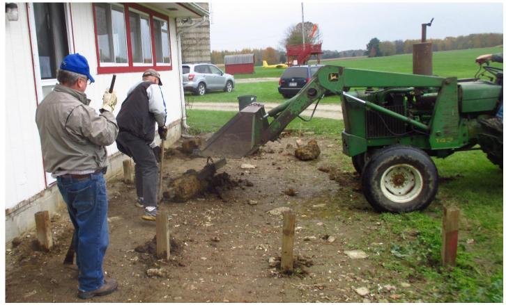
The rest of the crew pitched in to remove rusted bolts. After they were cut with an abrasive wheel the bolts were hammered out with punches. Boards were pried loose with spud bars and 4 X 4 posts were pulled with the tractor. Some of the 4 X 4s were in cement.
