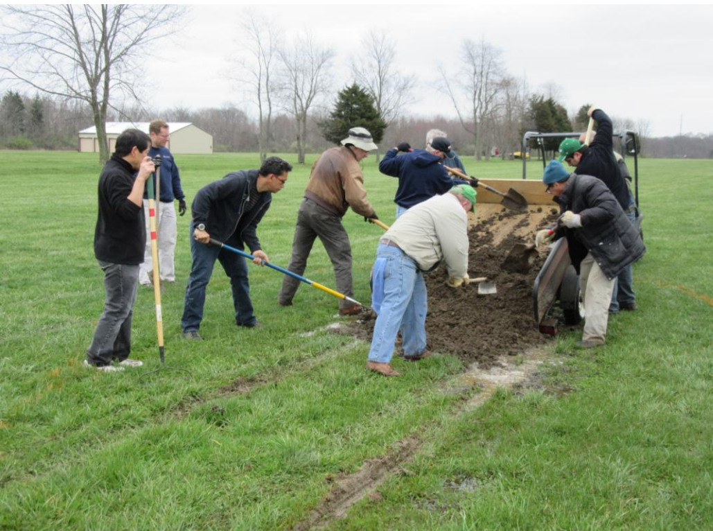
Once Steve Statkus had maneuvered the trailer to the location of a hole in the runway the crew made quick work of emptying the trailer. Photo: JCD
