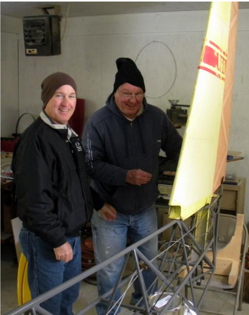
Keith Kilpatrick and Ron Kellerman fit the vertical stabilizer into place and check the length of rudder cables to assure everything is ready for covering to commence.
