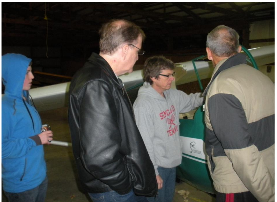
Tim Morris takes a break from his annual inspection of 135 to explain repairs that he, Keith Kilpatrick and Steve Statkus completed to return it to an airworthy condition.
